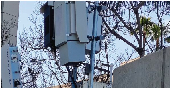
Figure 3.12 Pictorial illustration of a Qualcomm® remote radio head with a 32 \times 4 dual-polarized array.
